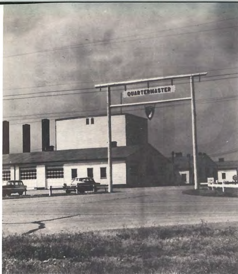
Parachute Maintenance Building.
