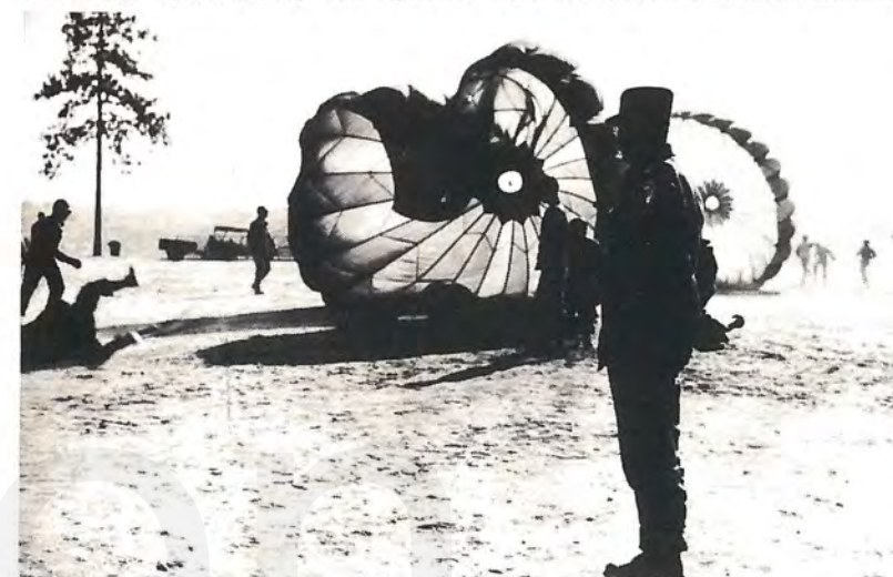
187th ARCT fledgling paratroopers learn the technique of making a parachute landing by controlled drop from swing trainer. Rakkasan in harness will be released by instructor holding rope, right. U.S. Army Photo
