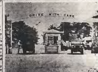
IT KEEPS THE RAIN OFF—Recently completed at the Camp Chickamauga main gate, this sign and use MP next went into immediate service at the Camp
