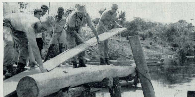
The Assault Pioneer Platoon repairing the landing stage at Tacama. Rfn. Coyne, Cpl. Fendyke and Sgt. Horsley.
